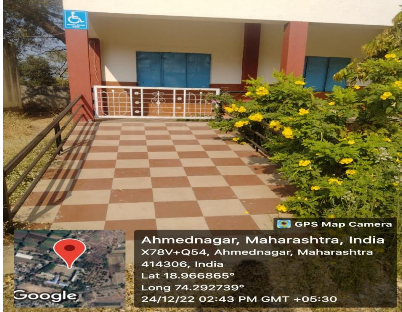
Photograph of Ramp for (Divyangjan) students to easy access to classroom
