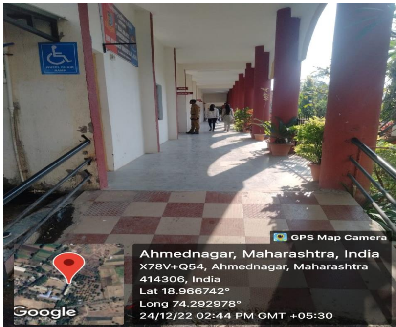
Photograph of Ramp for (Divyangjan) students to easy access to classroom
